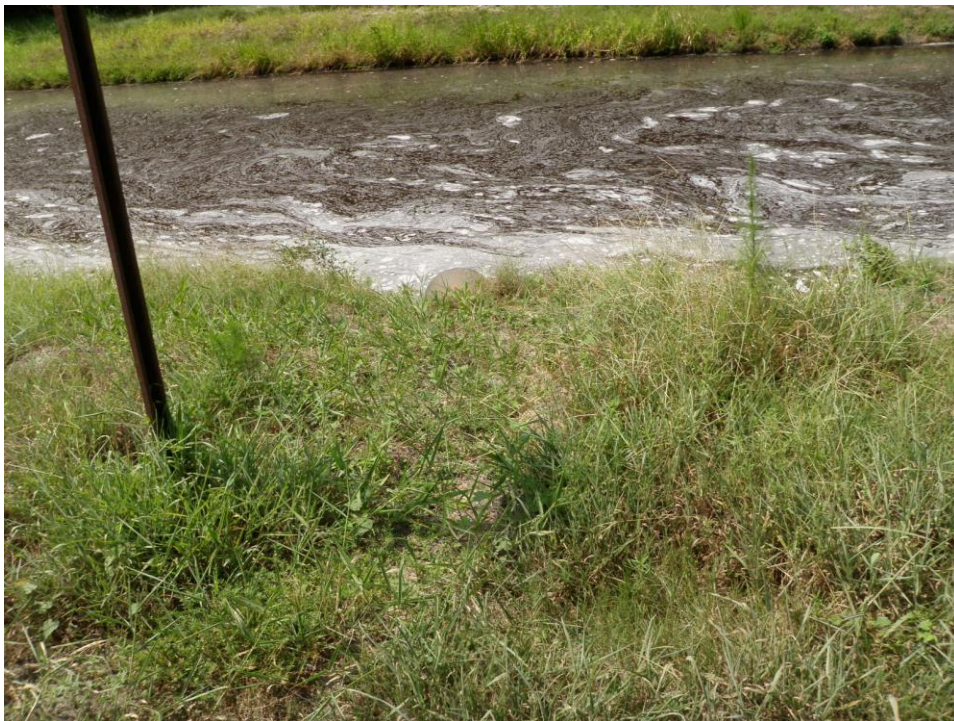
City of Crossett wastewater pipe discharging into GP system
