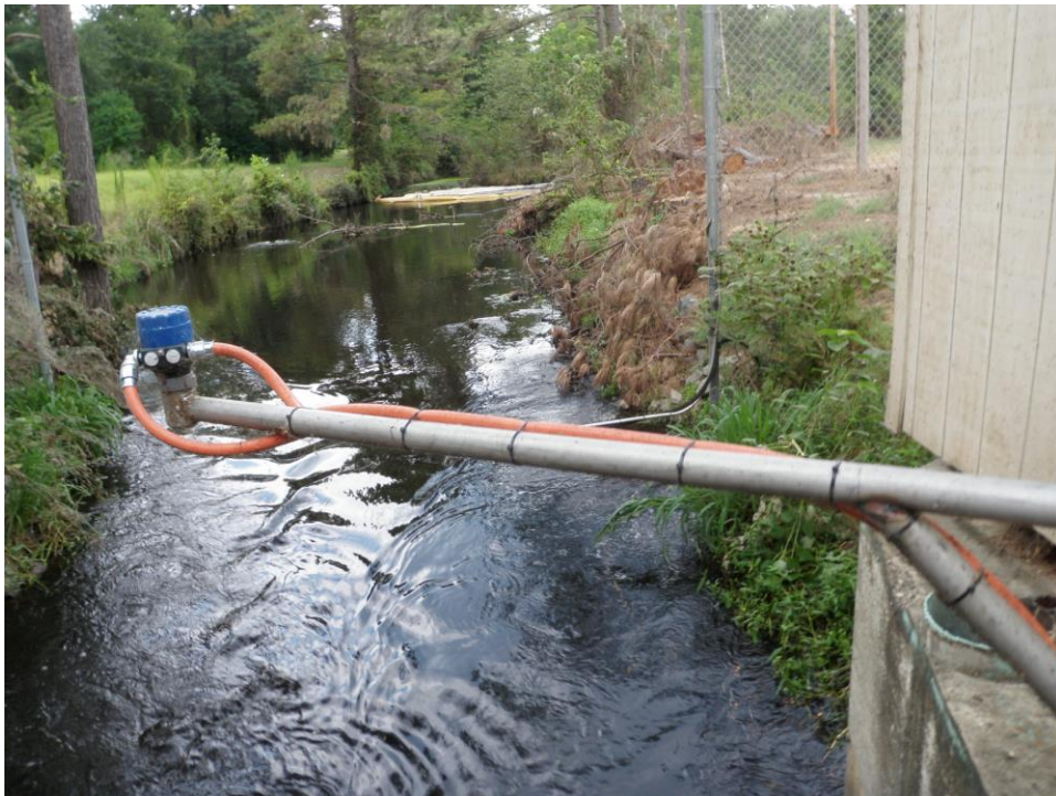
View at defoamer addition looking towards ASB and foam curtain
