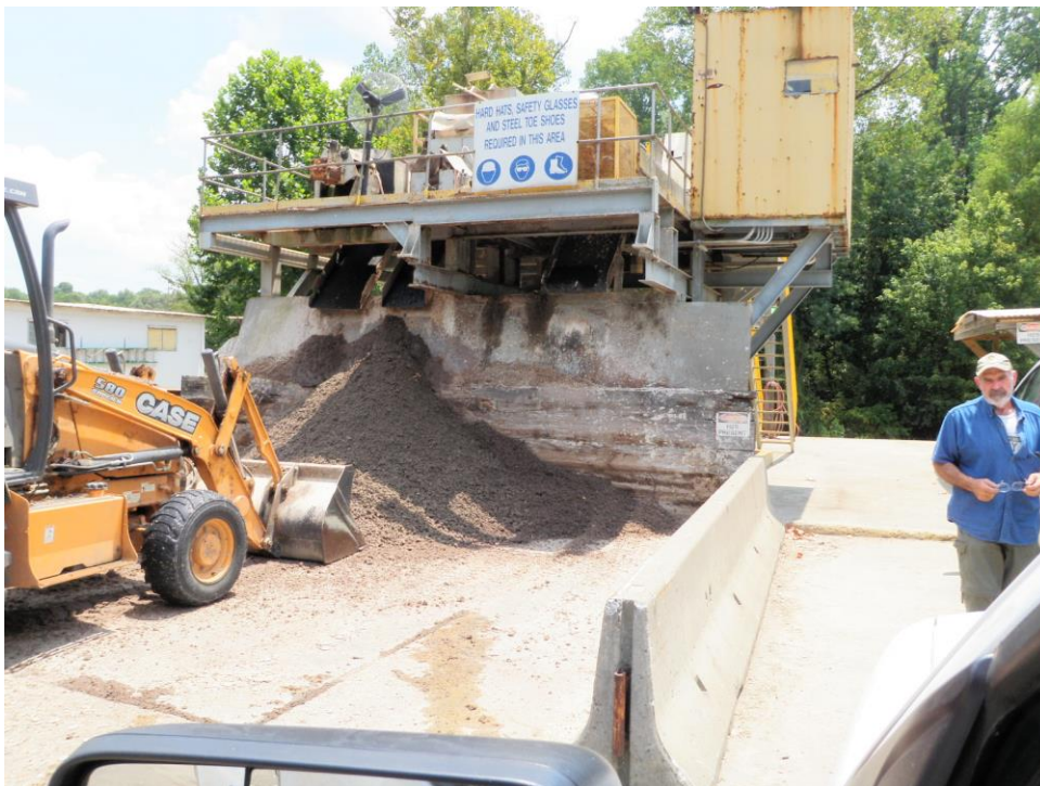
Dewatering of solids from the clarifier
