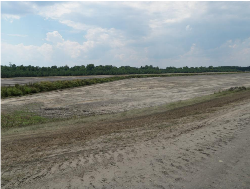
Empty Surge Basin
