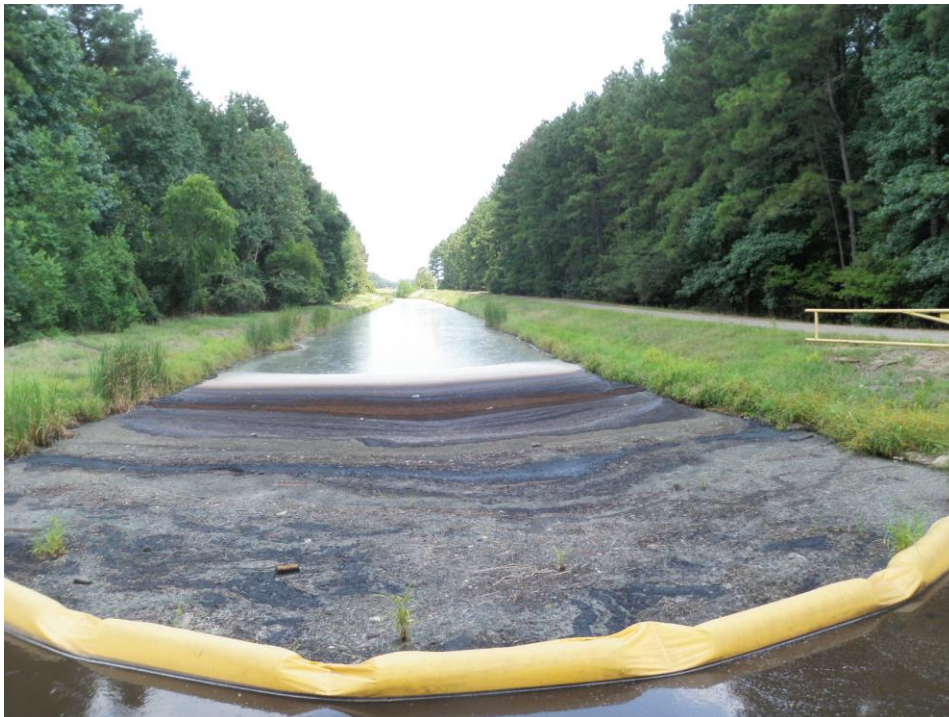
Channel from Surge Basin to ASB
