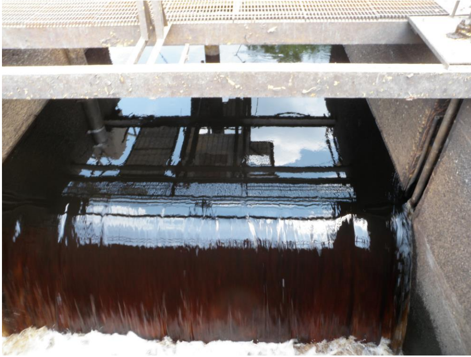
Outfall 001 – effluent flowing off the edge is causing foam to appear in the stream but the foam quickly dissipates.
