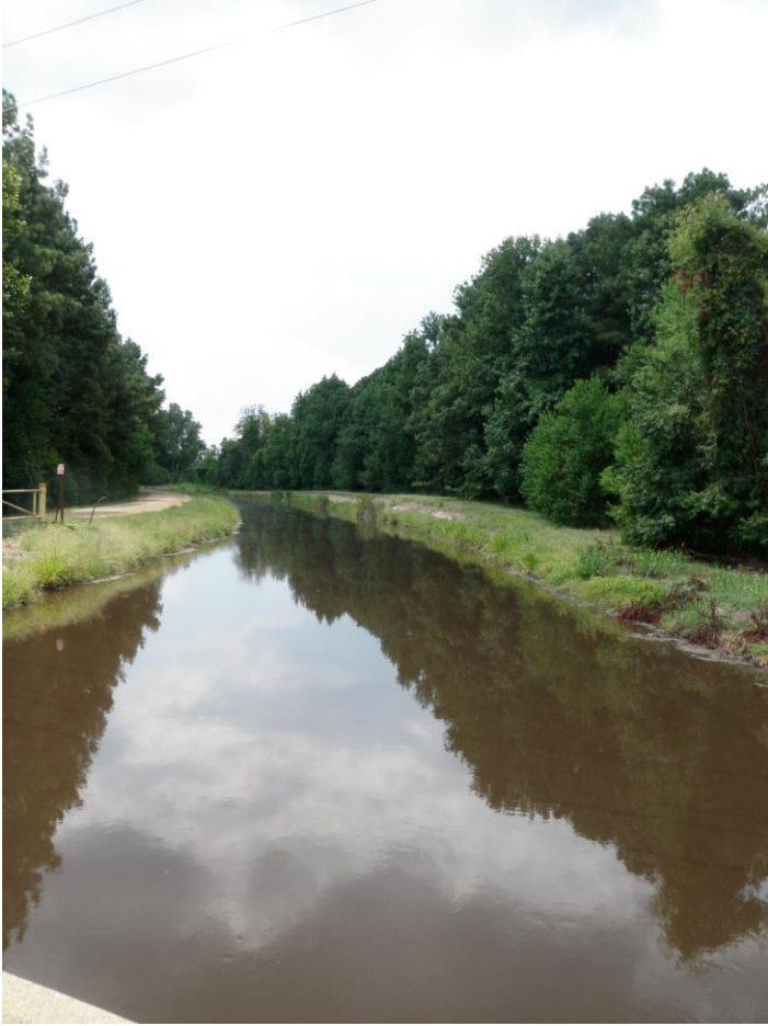
Surge Basin Channel looking towards ASB
